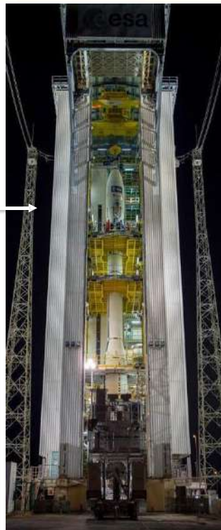
Mobile Gantry Launcher Integration
